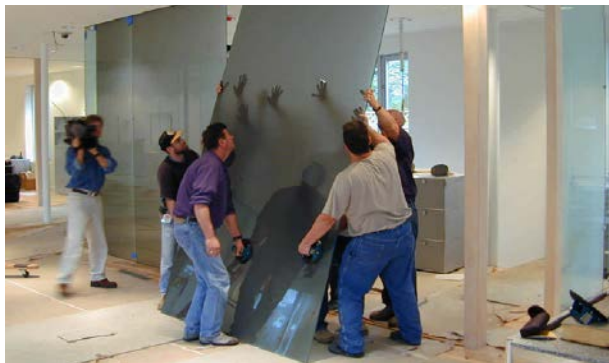
Installation of transparent glass panels
